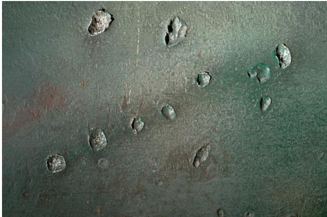
Figure 6. Bullet and shell fragment scars to side of the tank [2]
